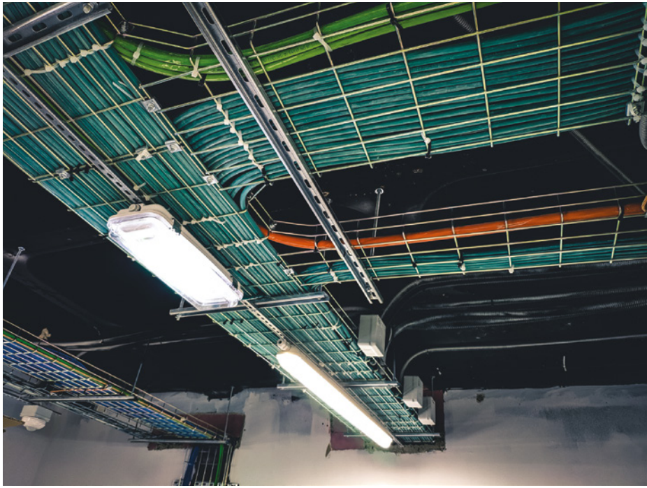
FIGURE 11.3 Cable distribution runs
